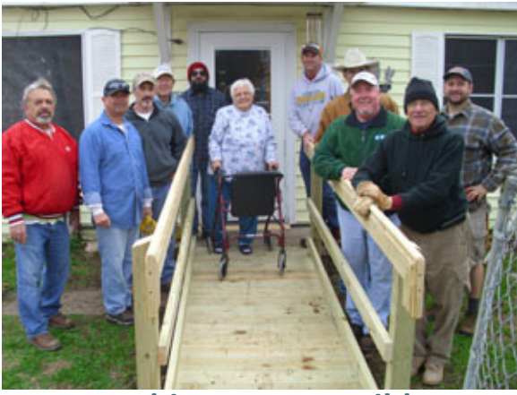
Habitat Ramp Build January 21, 2012
